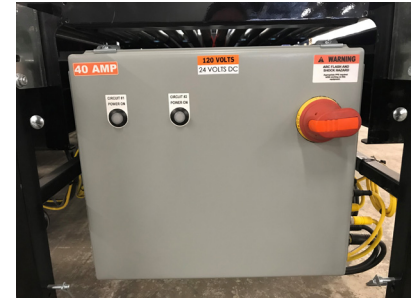
Figure 7: Power Panel with Disconnect Switch
